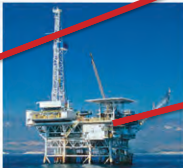
API rated Crane winches on Offshore Production Platform
