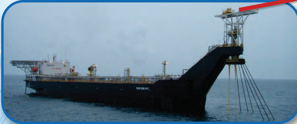
Swivel, Riser & Mooring Line Handling Winch on FPSO – SOFEC
