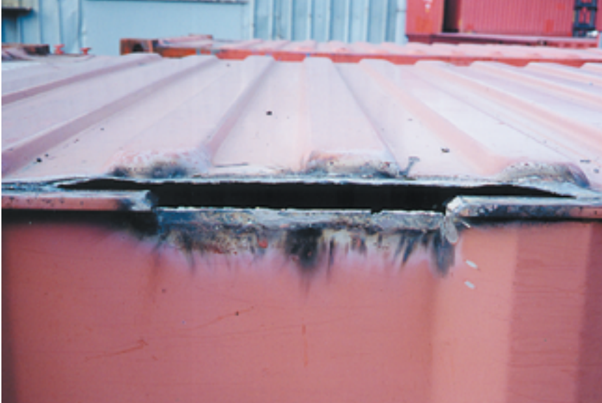
Photo 5.2 (to right) / Flat-bar top side rail section installed before welding, showing beveling of section and original rail to a combined 60 angle
