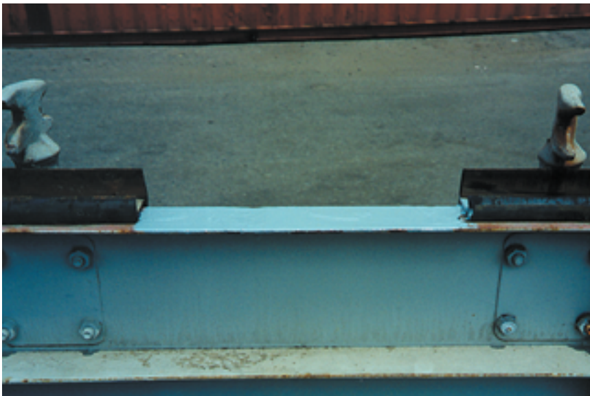
Photo 10.7 (to left) / Primed area of door under gasket
