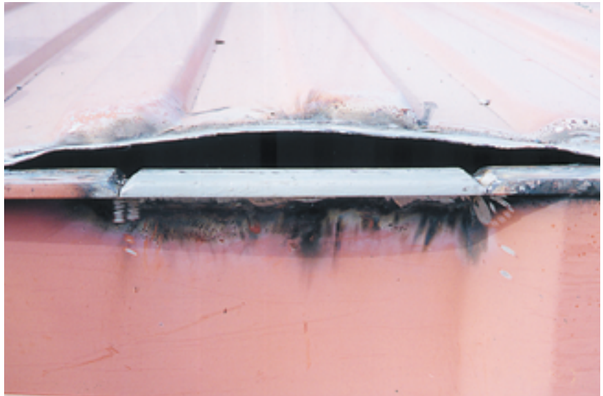
Photo 5.2 (to right) / Flat-bar top side rail section installed before welding, showing beveling of section and original rail to a combined 60 angle
