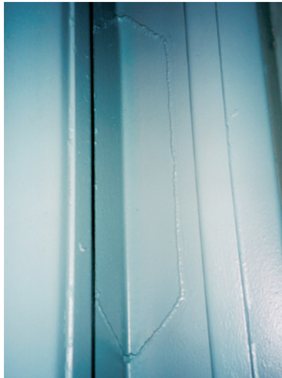
Photo 4.3 / Front corner post insert not adjacent to corner fitting (interior view)
