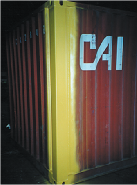
Photo 2.28 / Priming of replacement front corner post
