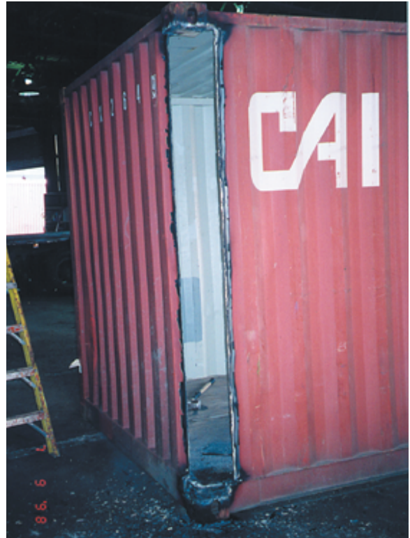
Photo 2.22 / Removal of corner post showing cut edges ground smooth
