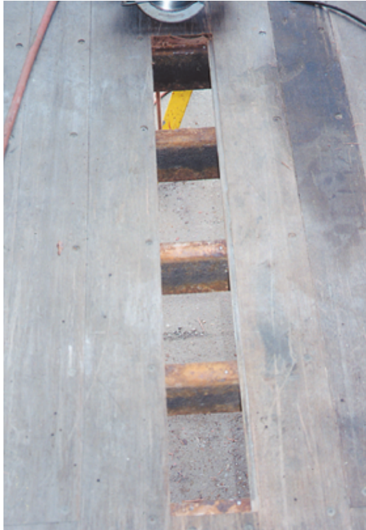
Photo 9.2 (above) / Removal of damaged section from a plank floor
