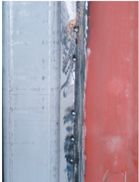
Photo 2.24 / Tack welding replacement front corner post in position
