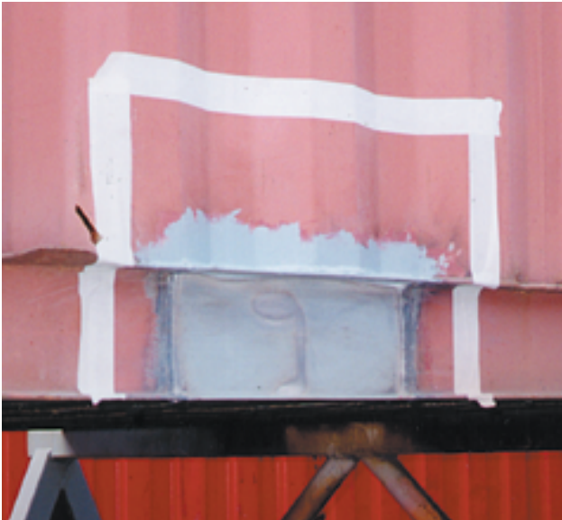
Photo 2.31 / A section repair to a bottom rail has been squared off with masking tape and priming has begun.
