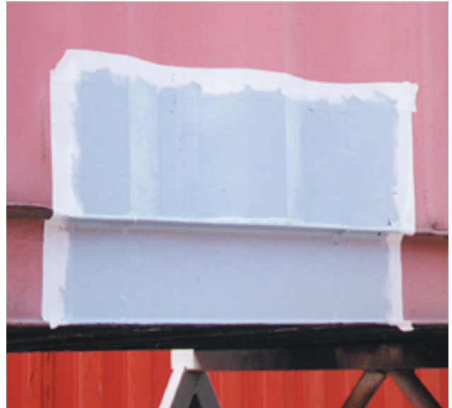
Photo 2.32 / The same repair, with priming completed within the masked-off area.
