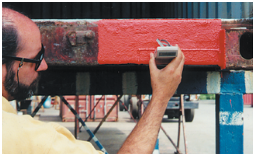
Photo 2.33 (to left) / Top coating of bottom rail section completed.
