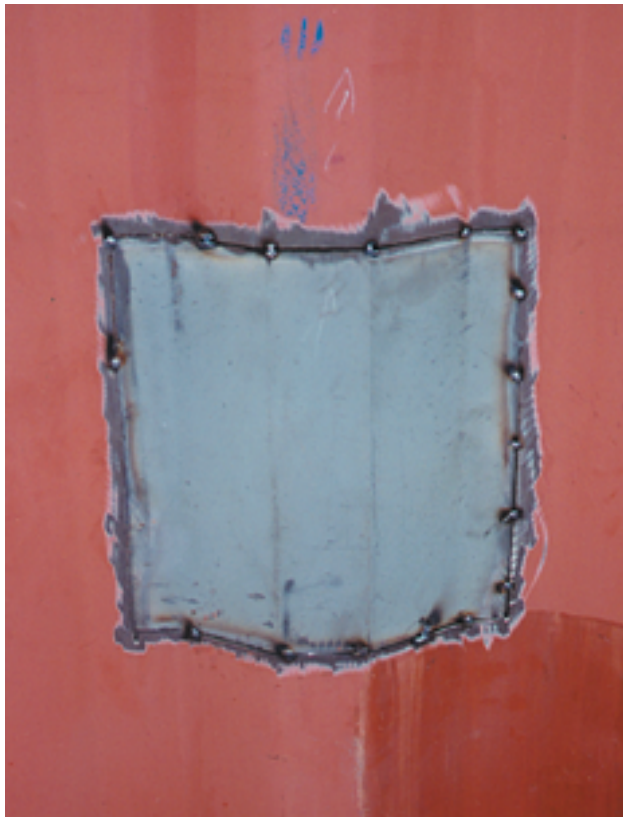
Photo 2.7 / Panel insert tack welded in position
