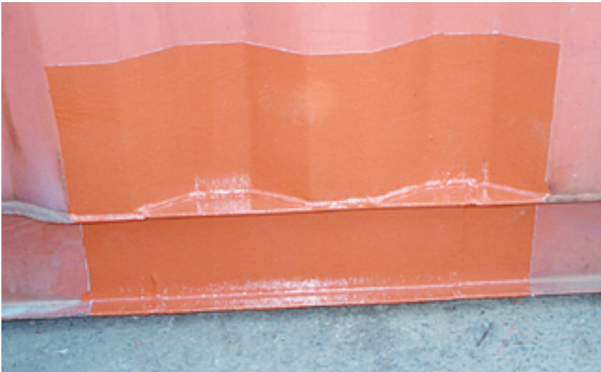
Photo 2.31 / A section repair to a bottom rail has been squared off with masking tape and priming has begun.
