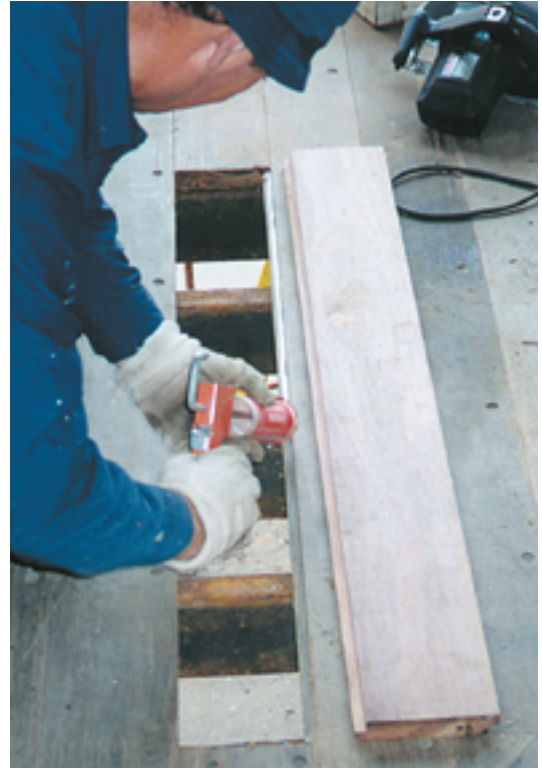
Photo 9.6 (above) / Application of sealant along shiplap of adjacent plank
