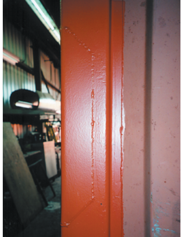
Photo 4.2 / Front corner post insert not adjacent to corner fitting (exterior view)
