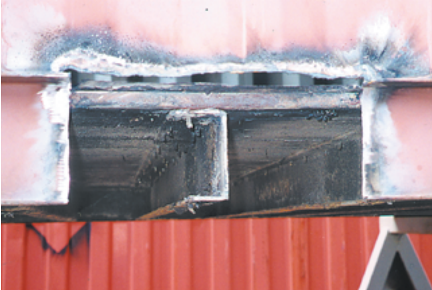
Photo 5.8 (to right) / Welding of bottom rail section to original rail, panel and crossmember
