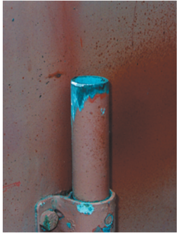
Photo 10.2 / Cleaned, smooth, beveled cut edge of locking bar
