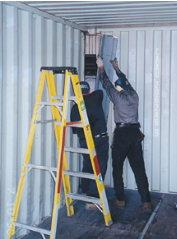
Photo 2.23 / Fitting a replacement corner post into place
