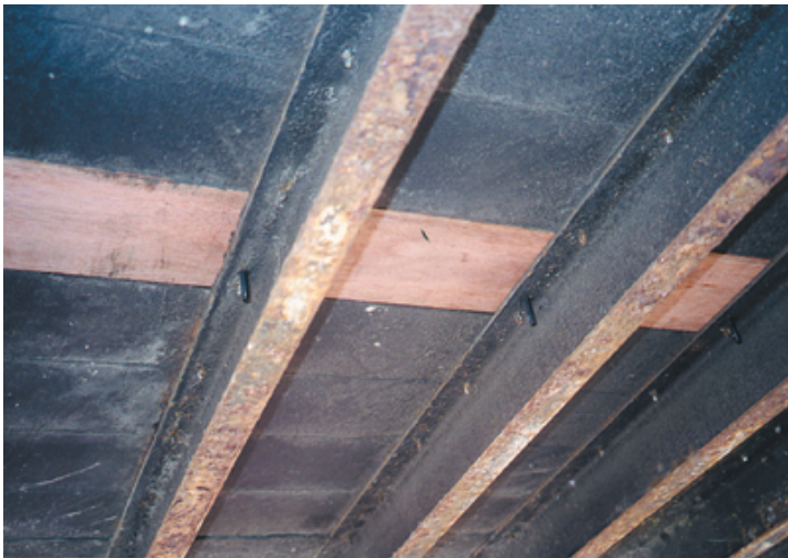
Photo 9.11 (above) / Screws installed into new plank section, fully engaging flange of crossmember (underside view)
