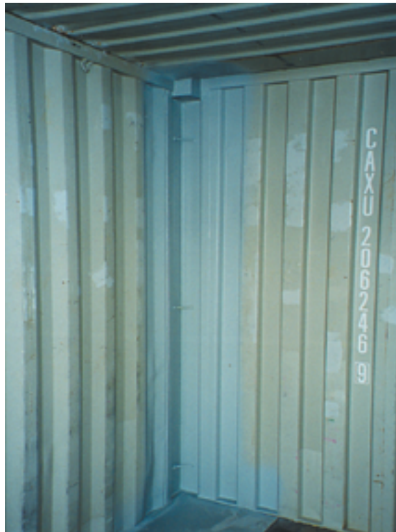
Photo 2.30 / Top coating of replacement front corner post (interior)
