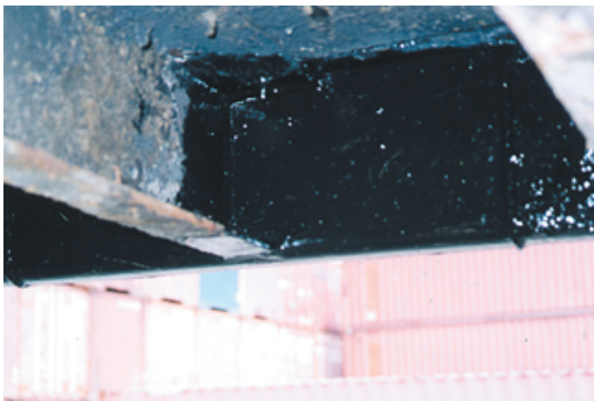
Photo 5.9 (to left) / Undercoating bottom rail section (primer was applied beforehand)
