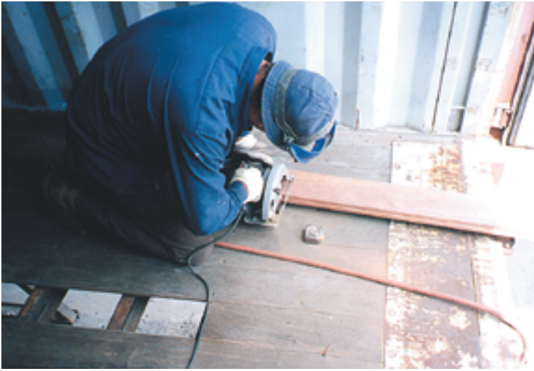
Photo 9.5 (above) / Cutting a plank to fit damaged area
