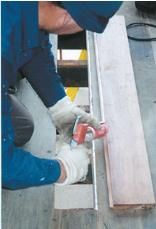
Photo 9.7 (above) / Application of sealant along shiplap of new plank section
