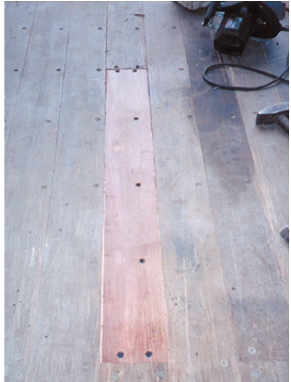
Photo 9.10 (above) / Screws installed into new plank section (interior view)
