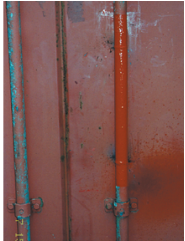
Photo 10.4 / Replacement locking bar section completed, including top coating
