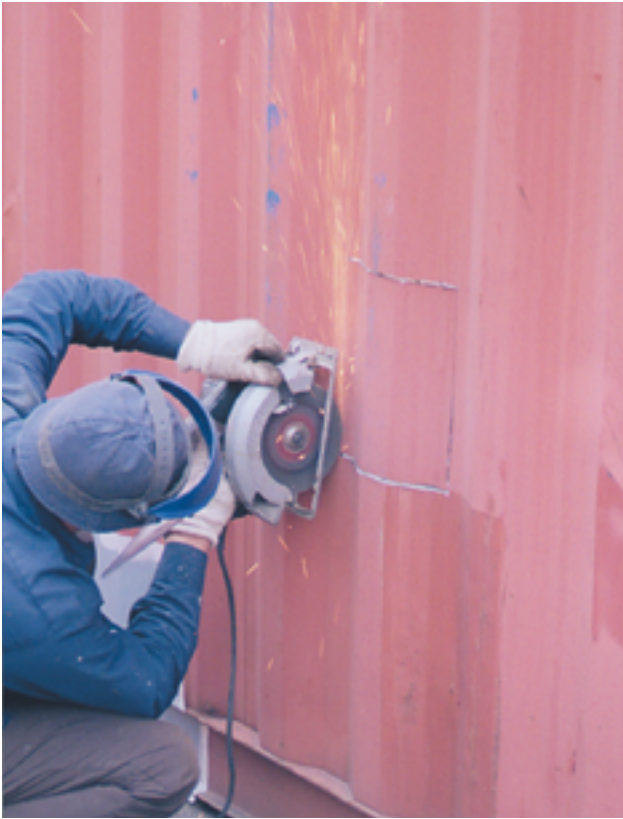
Photo 2.5 / Removing a portion of panel using a disc cutter (disc grinder)
