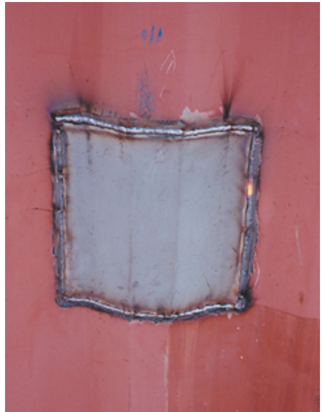
Photo 2.8 / Panel insert continuously welded
