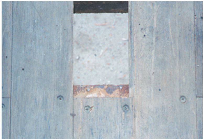
Photo 9.3 (below) / Plank floor joint lying above center line of crossmember flange
