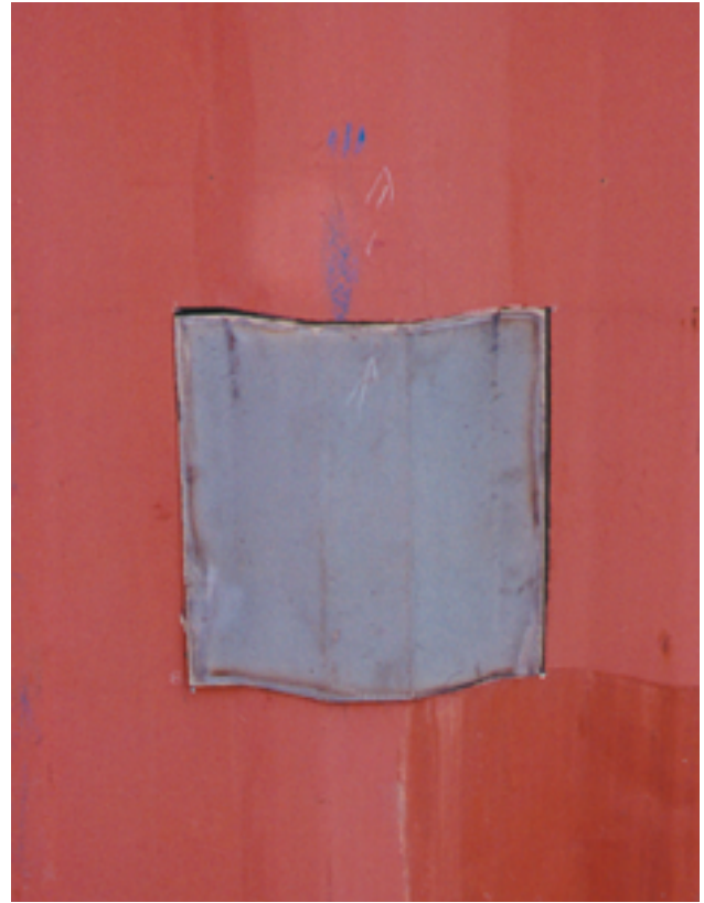
Photo 2.6 / Panel insert fitted into place (before welding)
