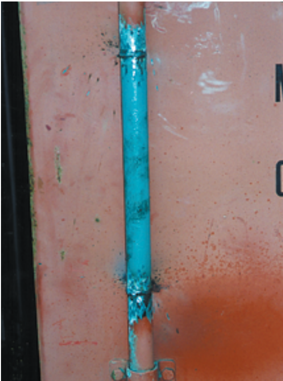
Photo 10.3 / Replacement locking bar section continuously welded in place
