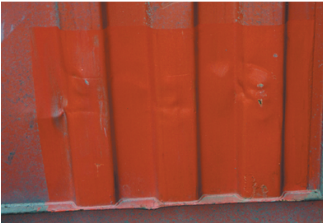
Photo 6.2 / Example of fair panel straightening, with fair corrugation profile and more serious hammer marks
