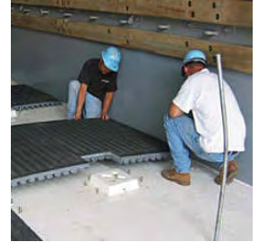
BATTERBOARD AND SYNTHETIC DECKING Batterboard and Decking for Well Deck
